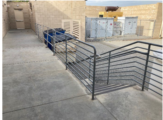
Trash Dumpster with Railing
